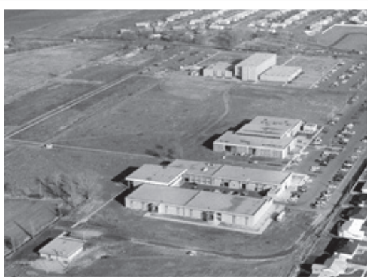
Aerial photograph of the Redwood Campus of Utah Technical College at Salt Lake (Salt Lake Community College) as it appeared in 1970.
